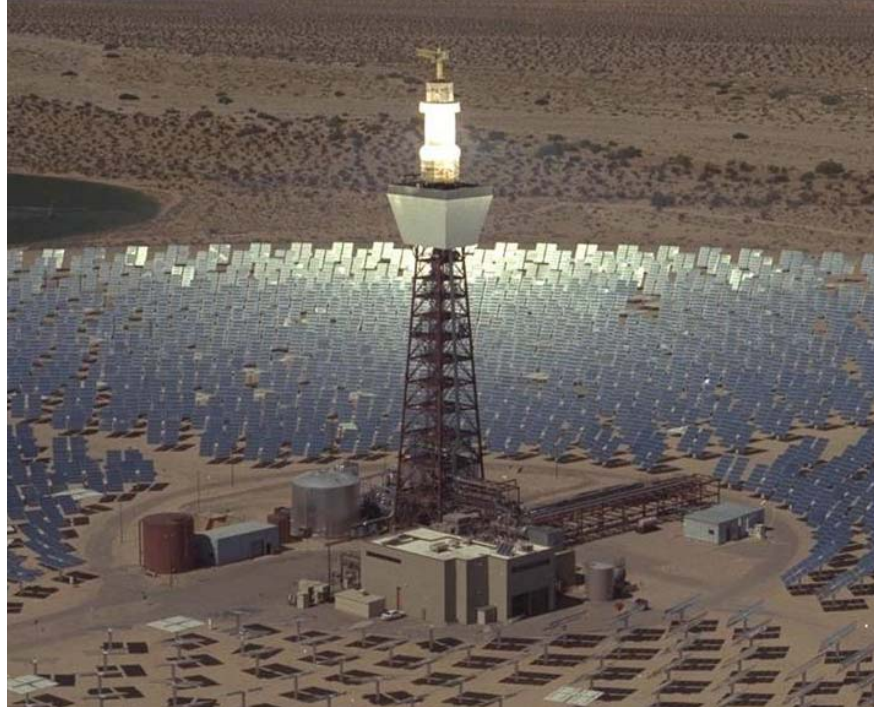
Figure 3. Photo of Solar Two power tower plant in operation in Daggett, CA (photo from Sandia National Laboratories, photo 2897).
