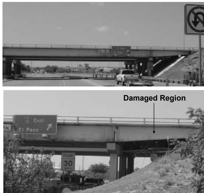
**Figure 10-1: I-10 Bridge at Avenida de Messilla in Las Cruces, NM (Westbound Lanes); Damaged Area is Indicated in the I-Beam Directly Under Westbound Traffic**
